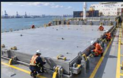
Hatch-cover seal inspection
